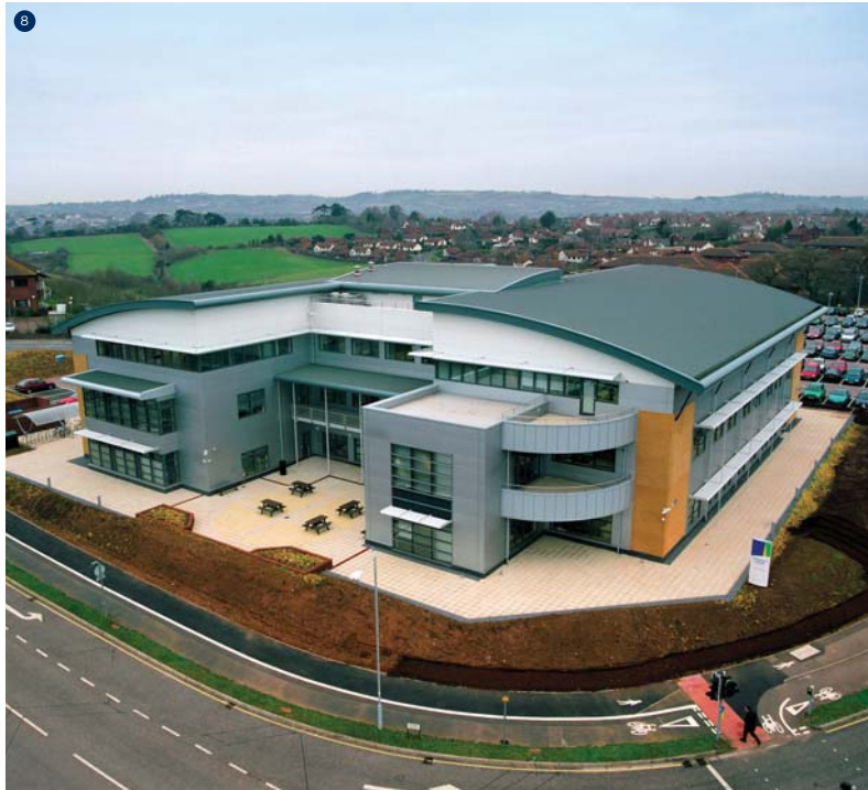
8 Norwich Union Headquarters, Exeter Architect: Ian Penrose, Exeter Cladding Contractor: Progressive Systems Ltd
