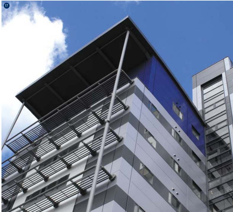
17 Mill Street Student Accommodation, Leeds Architect: Halliday Clark Cladding Contractor: County Cladding
