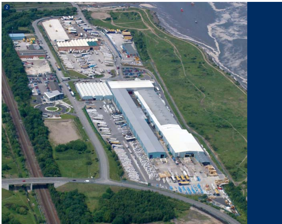
2 Kingspan Insulated Panels Holywell site in North Wales
