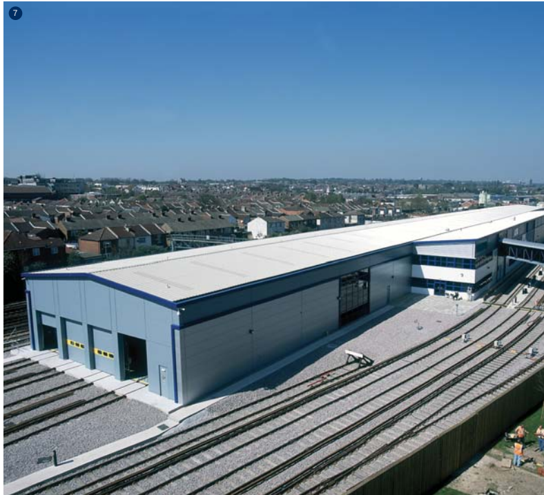
7 Siemens Traincare Facility, Southampton Architect: Burks Green Contractor: Fitzpatrick
