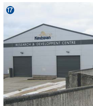
17 Kingspan's R&D Centre in Kingscourt, Ireland
