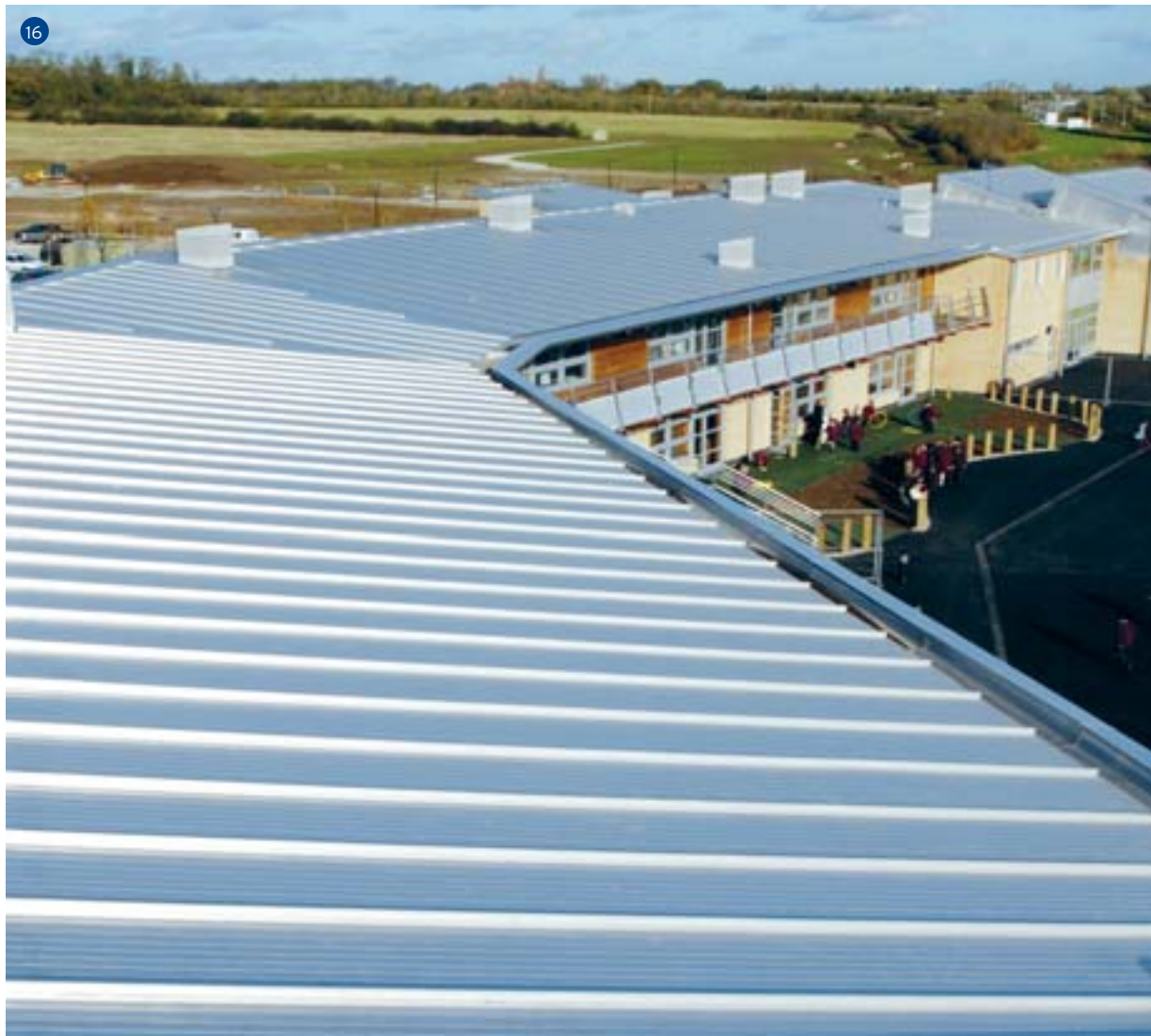
16 Oxley Park School, using Kingspan's Kingzip standing seam insulated panels
